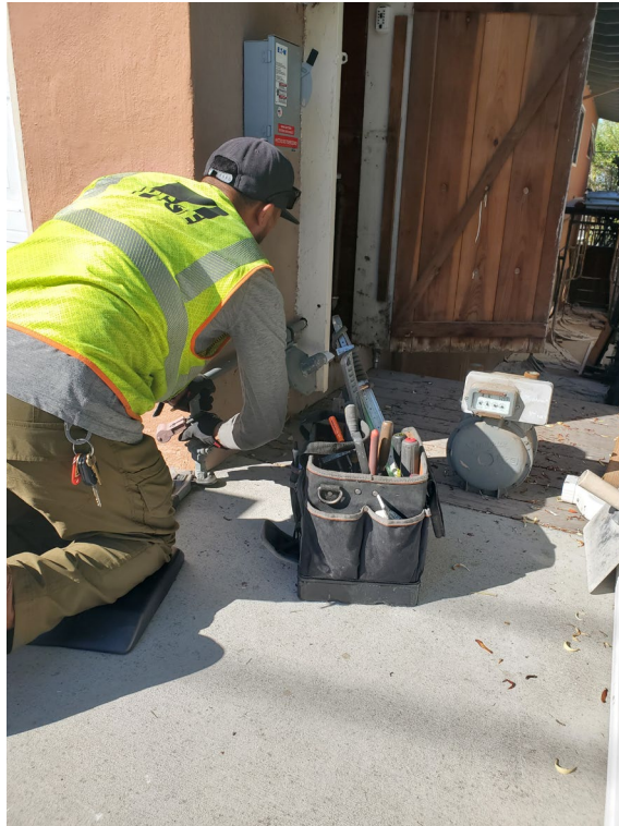
Removing natural gas meter, August 2022.
